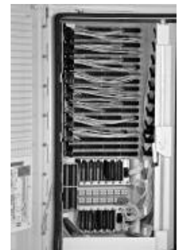
OptiText Premier Cabinet (432 fibers) with Splitter Module Detail | Photo HWPSS1751
