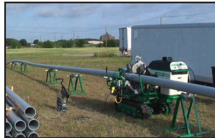
Example of fusion machine setup at jobsite
