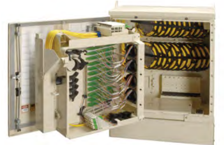
Ground Mount Small 288 Configuration with In-Hub Distribution Cable Splicing
